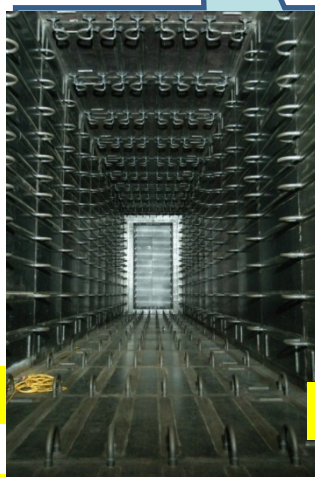
Decay volume completed
