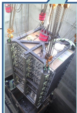
Beam dump completed
